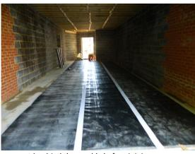
surfaces must be dried thoroughly before joining.
